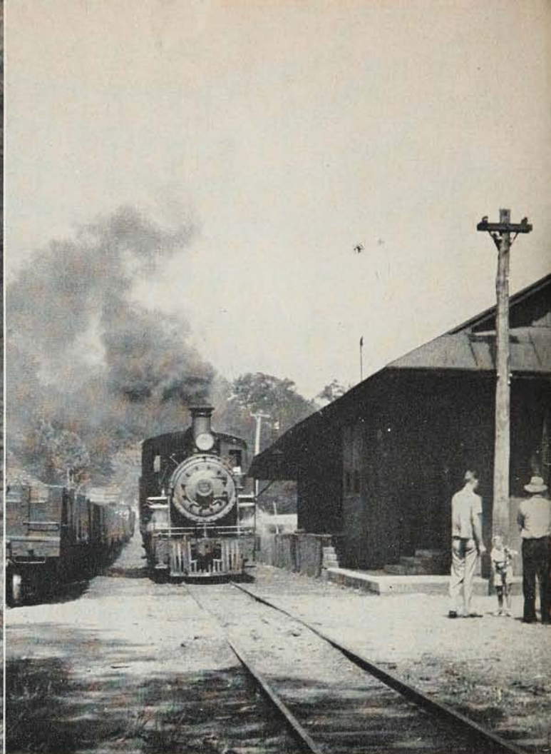
No. 11 rolls to a panting stop at Elk Park, N. C., after a hard climb up the 3 per cent grade from Elizabethton, Tenn. A few of the townsfolk have turned out to greet the train in true country tradition.
