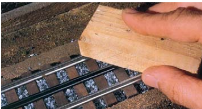
4. Gently tapping along the rails with a block of wood spreads ballast under rails and imparts a slight crown. Be sure to fill any low spots with more ballast.
