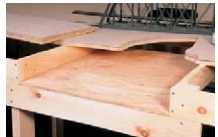
Fig. 2: Next you frame the gorge the same way that Stan did — with 1-by-4 sides and a base made of plywood. Be sure that they fit flush to the front edge of the layout.
