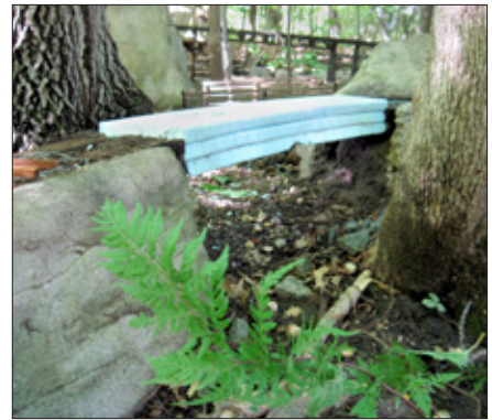
3. Working from the top down, each new layer is glued to the one above.
