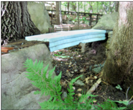
4. By cutting increasingly larger sections out of the middle of each new layer, the bridge's arch takes shape.
