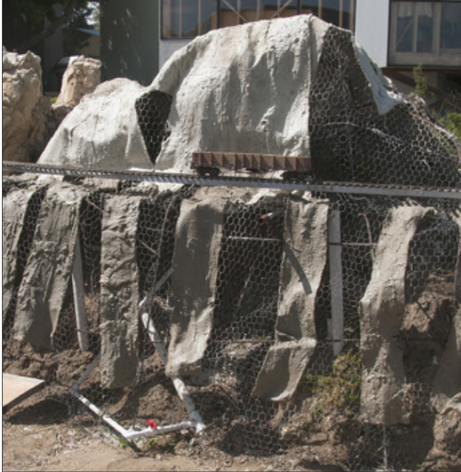
8. Mountain construction techniques changed in the rebuilding of the line. Cement-soaked burlap was placed over chicken wire and rebar to support molded-cement rock slabs. An aluminum-and-PVC spline supports the track separately from the scenery.
