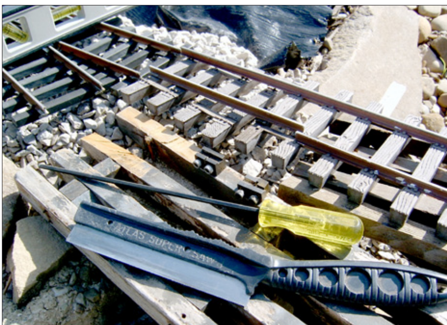
A section of rail is being inserted between the track and a turnout to fill the gap in the outside rail produced by a long curve. Two Split-Jaw Rail Clamps and a ball end, Allen-headed screwdriver are in the middle.
