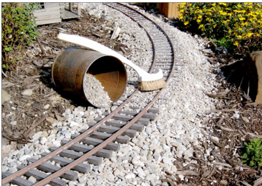
Adding ballast (#9 crushed limestone) over the #8 limestone roadbed. A can and an old dishwashing brush facilitate the process.
