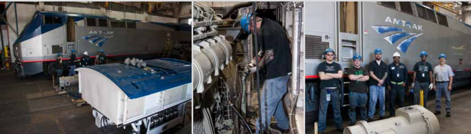
No. 90's new roof hatch from Beech Grove goes on after the motor is installed, left. Above, machinist Tom Shriey connects the motor to other systems. Right, the Chicago crew that did No. 90's engine change out pose with their million-mile project. Six photos, Bob Johnston
