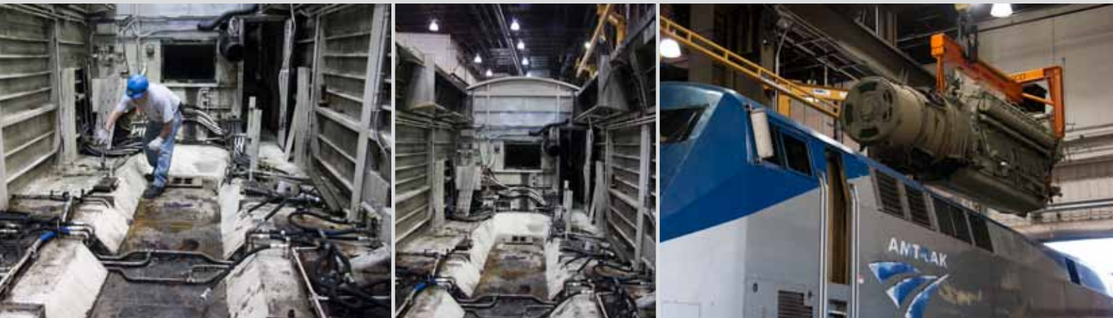
With components removed, Romero Gutierrez prepares the engine room for the replacement 7FDL16 power plant. The interior is full of cabling and hoses to connect all systems. A crane carefully lowers the alternator and diesel engine into the carbody on June 7, 2012.
