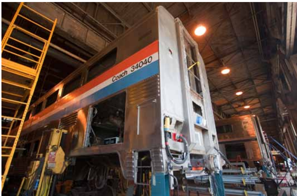
Superliner I coach 34040 survived the 1993 wreck of the Sunset Limited , but had to wait 17 years for extensive structural repairs, new wiring, and a complete interior makeover.
