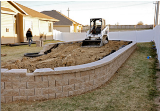
C. Installation of the wall blocks is nearly finished.
