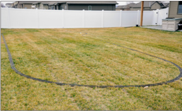
A. Track was laid on the ground so the landscape crew could get overall dimensions of the railroad and curve radius correct. They did a beautiful job; the track fits against the lip of the wall perfectly.
