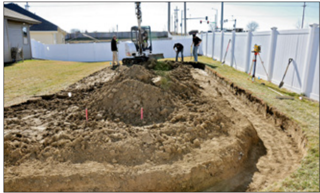
B. The big dig is under way for the foundation gravel.
