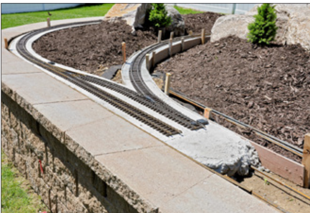
E. Some of the concrete roadbed has been poured. Rebar is used as reinforcement.
