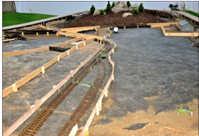
D. Concrete forms for the roadbed, parking lots, and streets are in place. White PVC pipe provides an electrical access point from the house to the railroad.
