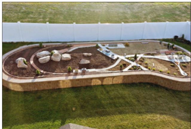
F. The nearly finished railroad. Trackwork has yet to be completed.
