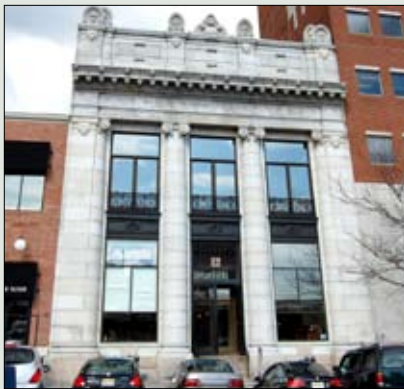
A. This is the original photo taken of the Trust Company of New Jersey building. Notice that it is distorted, converging toward the top. While this photo is useful as a general view, it is not very useful as a pattern for making plans.
