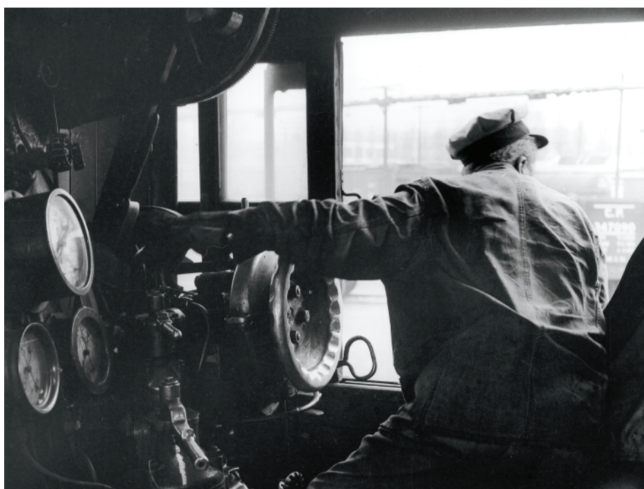
Another April 27 view of No. 2826 shows a hostler moving her around The Glen. The big "steering wheel" is in fact the control for the engine's air-operated screw-type reverse, common on newer CP power.
