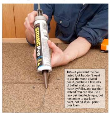
After the Liquid Nails dried, we used brown acrylic caulk to hide any seams and fill any gaps between the foam boards. Once our foam-covered framework was done, we had a tabletop that already looked realistic, if a bit barren. At this point, the surface was ready for us to install track, which we'll cover next in our Build a Retro Railroad instructions.
