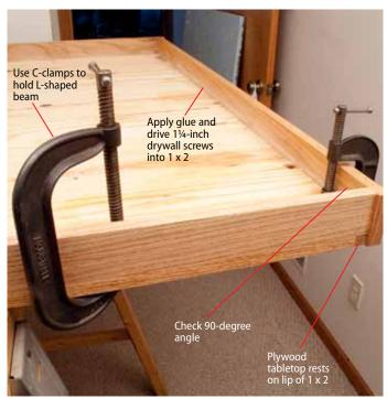
After allowing the glue to dry, we installed the L-shaped beams along the plywood edges. We used clamps to temporarily secure the 1  $\times$  2 lip of an 8-foot beam to the underside of the plywood. We confirmed that the 1  $\times$  3 fit at a right angle to the tabletop and then used wood glue and drywall screws to attach the beam.
