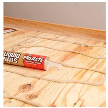
We used Liquid Nails For Projects brand latex adhesive (www.liquidnails.com) to bond the foam to the plywood. Bonding the foam to the plywood gives the plywood a little more strength. If you find that the foam wants to lift off of the plywood, use drywall screws to hold it in place while the Liquid Nails dries. You may remove the screws later.
