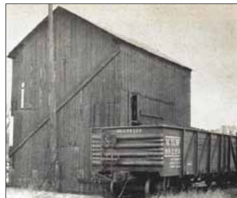
Prototype at Brodhead, Wis., was used to service locomotives on Milwaukee Road's Mineral Point branch. Coal was shoveled from gondolas through opening in rear of shed onto inside platform.
