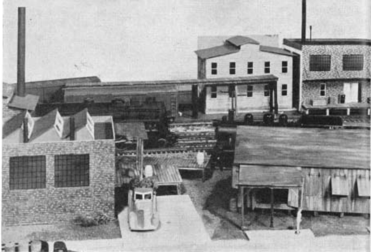
Vista between industries at Donaldson. The Hudson bulks powerful, pulling her string of varnish through town as the little way-freight's engine waits in the hole for the meet.
