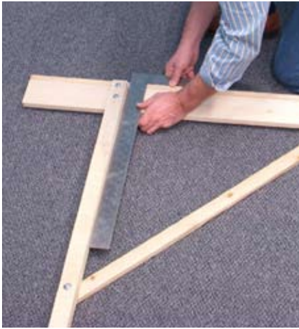
Fig. 2 Adding legs. The legs need to be absolutely perpendicular to the L girders for the layout to be stable. Here Stener is using a square to check the position of the legs.
