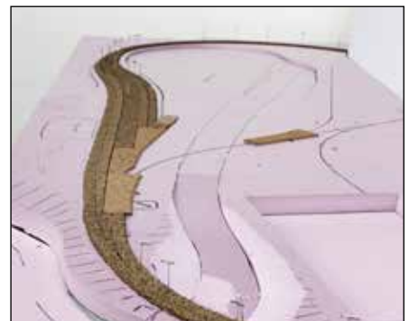
Fig. 17 Cork strips and pads. We used pre-cut cork pads under turnouts, but in other places we cut and fit cork.
