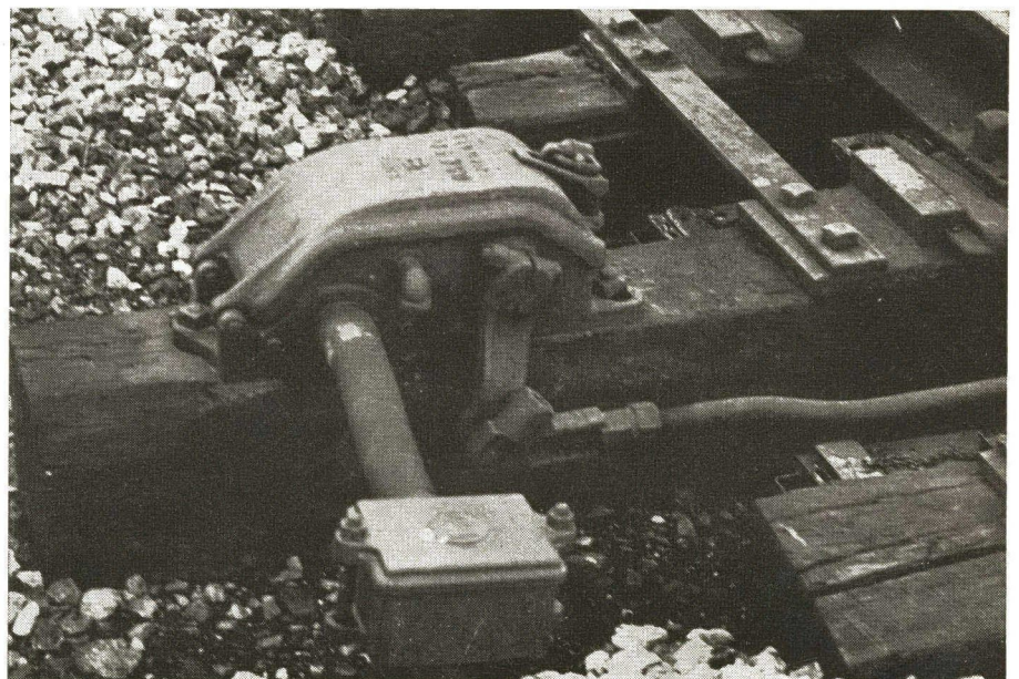
Upper left: Rodding at a turnout showing the connections to several components. From top to bottom: Dwarf signal for Hammond line, dwarf for Dolton line, turnout lock and turnout points. Above: Situation at a
