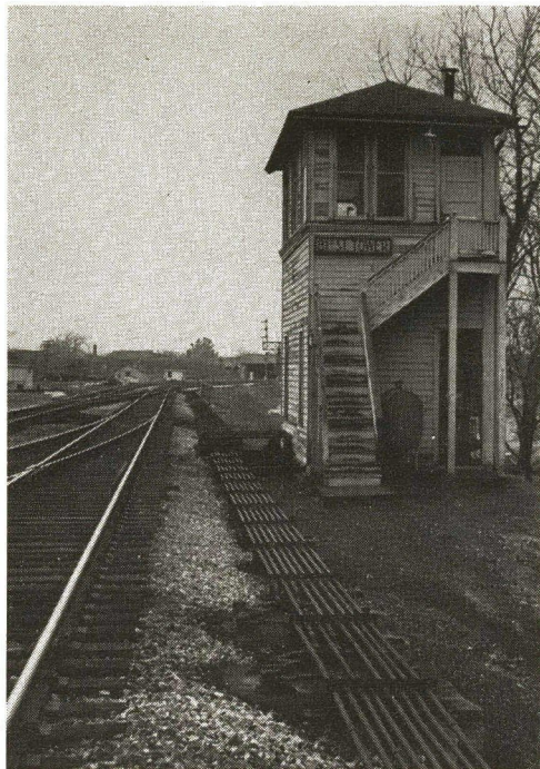
Chicago & Western Indiana's 81st St. Tower on Chicago's south side is a good example of a small, mechanically interlocked junction. Upper left: View toward the south past the single slip and the crossover. In the distance is the signal bridge with the automatic block signals on
