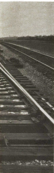
Chicago & Western Indiana's 81st St. Tower on Chicago's south side is a good example of a small, mechanically interlocked junction. Upper left: View toward the south past the single slip and the crossover. In the distance is the signal bridge with the automatic block signals on
