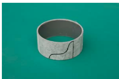
Lamp bracket marked out on a section of the tube used for the boiler shell.
