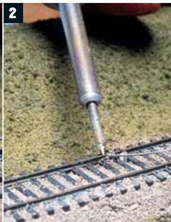
A Western Union splice is the preferred choice for end-to-end connections. Note the heat-shrink tubing to the right.
