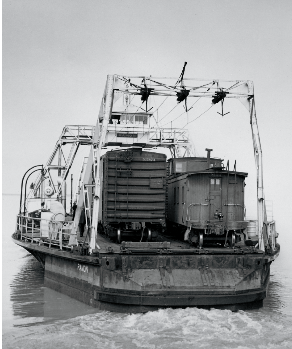
The Ramon , a 3-track ferry, moved cars between Mallard and Chipps. Because of the width of the cars, only two tracks are in use here. William D. Middleton photo
