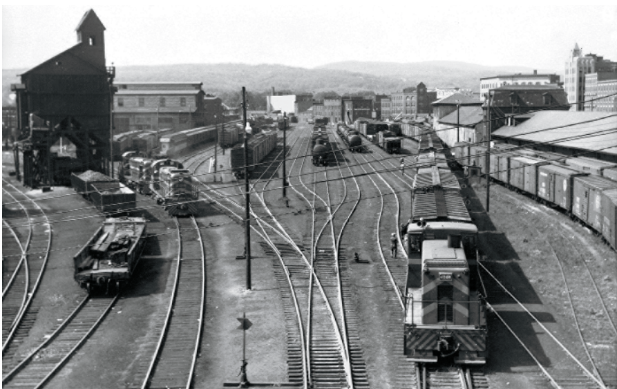
Fig. 11. W. Clifford Cottrell stood on the River St. overpass to photograph the Rutland yard in December 1954, two years after steam's demise. Looking southeast from
