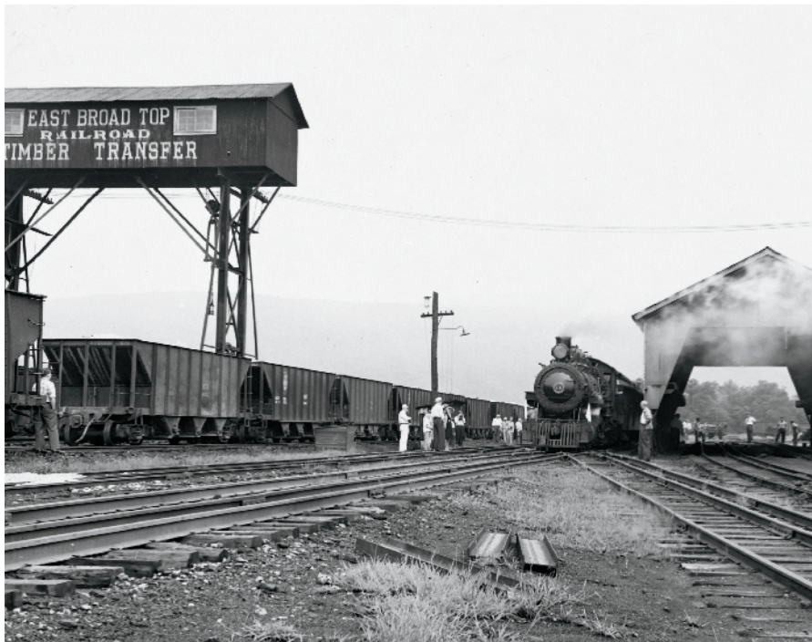
Figs. 21 (above) & 22. The East Broad Top brought raw coal to the preparation plant at Mt. Union, where it was dumped, cleaned, sized, and reloaded into standard gauge hoppers for shipment to customers via the Pennsylvania RR. The photo above was shot in 1953 by Philip R. Hastings. Near the prep plant was the old timber transfer crane, seen above and in the 1949 photo at left, which was taken by Charles S. Small. This crane was used to lift standard-gauge freight cars off their trucks, one end at a time, so narrow gauge trucks could be installed for travel over the three-foot-gauge EBT.
