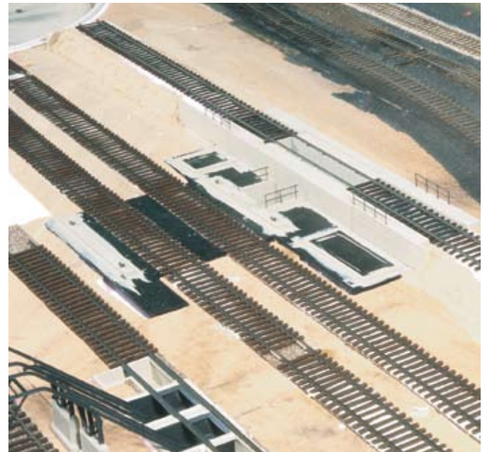
Fig. 9 Base. Here's the base worked into the layout and track laid. Bill made the tower and all the other structures so they could be lifted away to make layout cleaning easier.
