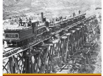
**28. SMALL LOCOMOTIVES, SHORT TRAINS:** The 4-4-0 and 4-6-0 locomotives of the Transcontinental Railroad era generally could pull 250-ton freight trains of 15 to 20 cars at an average 10 mph, or five- to six-car passenger trains of 90 tons at speeds rarely higher than 25 mph. UNION PACIFIC
